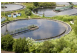
Mains Water Pressure Recording
